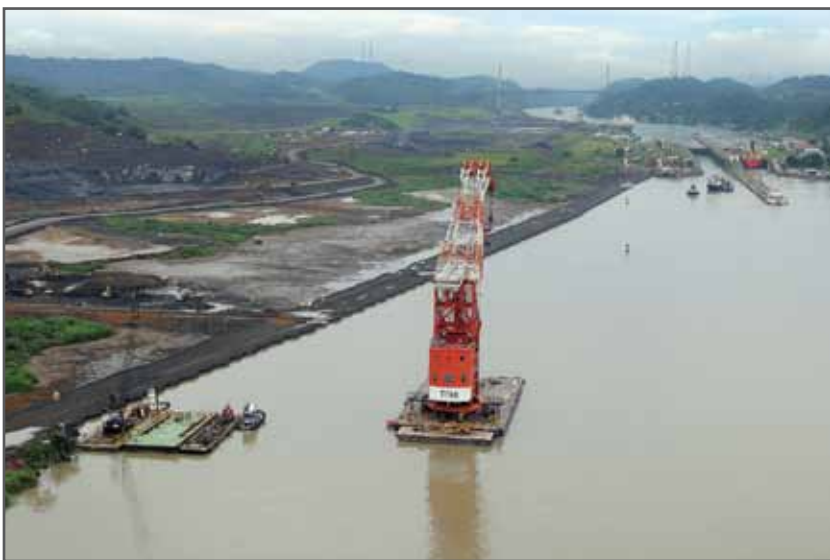
Borinquen Dam cofferdam
