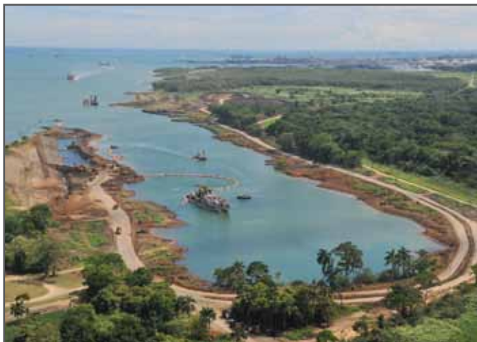
Dredging work on the Atlantic side
