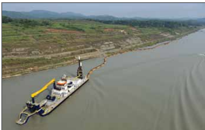
Dredging work at Culebra Cut - dredge Quibian I
