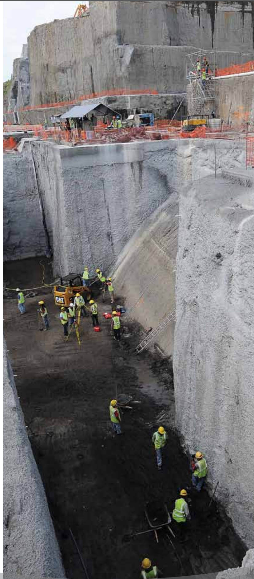
Work under the Atlantic locks project
