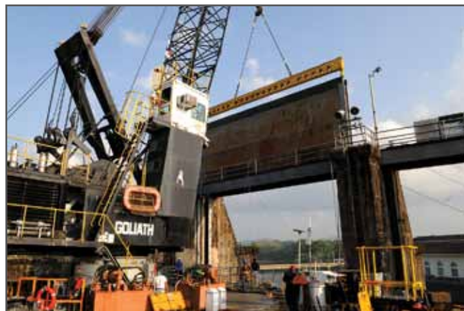
Modification of Gatun spillway gates
